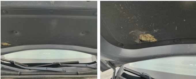
Front Bonnet / Insulation / Replace-tear
