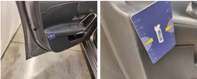
Front Left Door Interior Coating // Replace Completely-scratch
